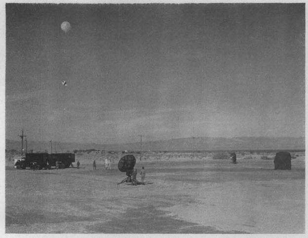
ALMOST LOST in desert wastes near Salton Sea is this mobile meteorological unit, shown making radiosonde observations on winds and air currents aloft. tion, to receiving instruments on the ground.
